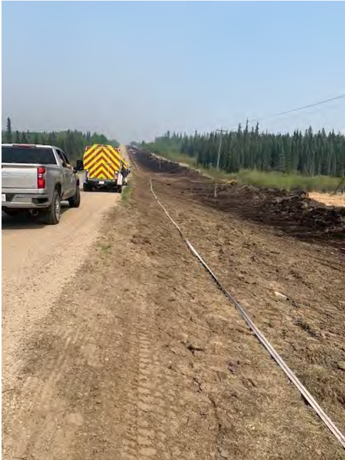
Sappers laid hoses for up to nine kilometres in length along the Virginia Hill Road to protect the town of Whitecourt, Alta.
