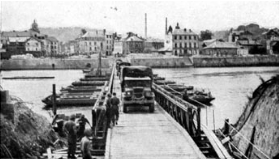
A pontoon bridge over the Seine in France – a Double Single Bailey
