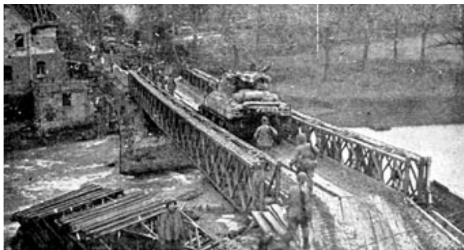
M4 tank crossing 110 foot Triple Single
