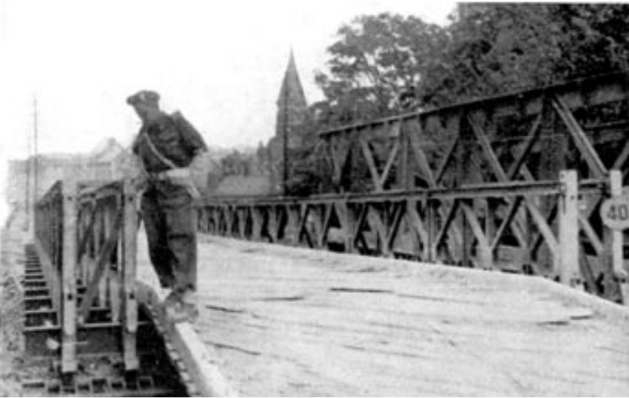
A Double Single Bailey bridge (over the Somme in France) see Appendix for bridge terms
