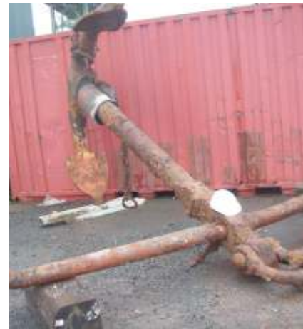
Lifting the anchor out of the ground (excavator bucket is approximately 2m wide). Anchors are manufactured for specific classes of vessel, by weight. Niobe was the only Canadian ship large enough to need this size anchor.
