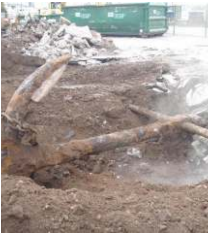
Each link of the chain weighs approximately 75 lbs (hard hat added for scale).
