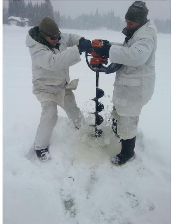
*Members from 51e squadron of 5 CER are drilling a hole through the ice layer that formed over Lake Hayes in order to install water pumps.*
