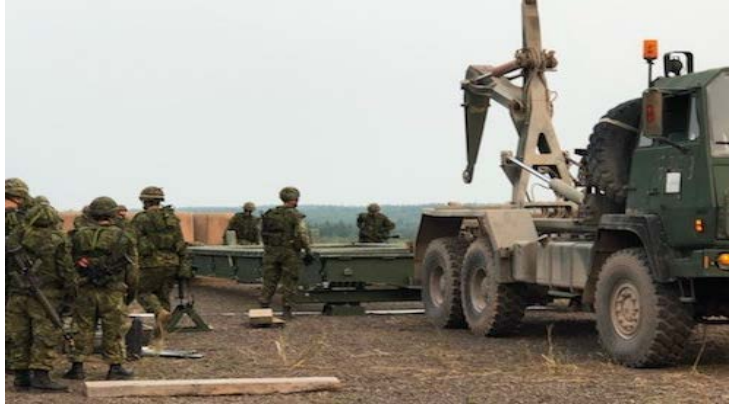
Members of 24 Reserve Troop rehearse bridge construction on Ex MAROON RAIDER 2018
