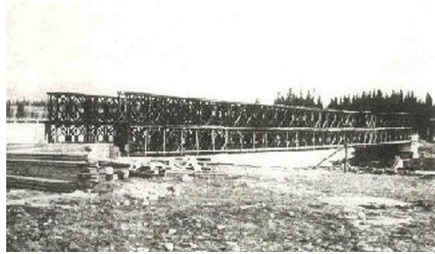
Kananaskis Bridge under construction
