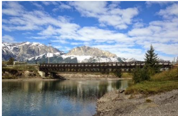
Kananaskis Bridge in 2016
