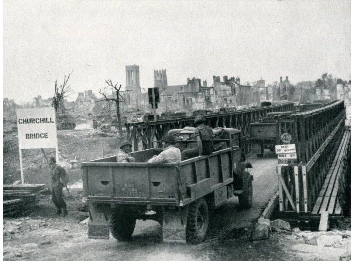
'Churchill' Bridge built by the 5 th Field Company, 18 July 1944
