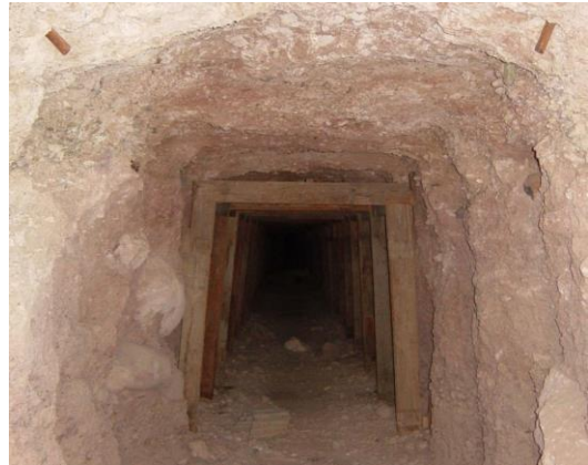
Tunnel with timber supports
