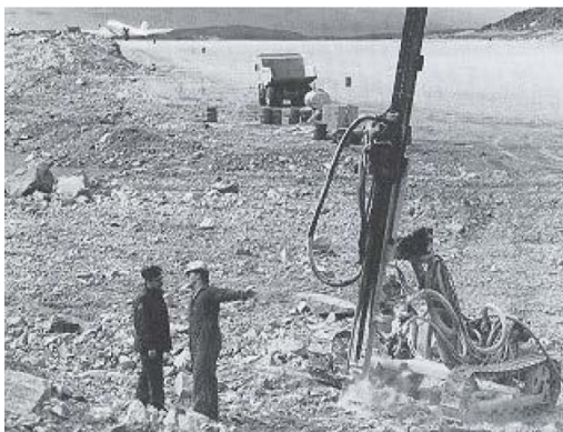
Northern airfield construction
