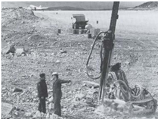
Northern airfield construction
