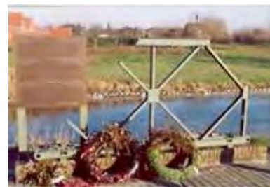
Figure 5-15 Sgt Hickman Bridge
