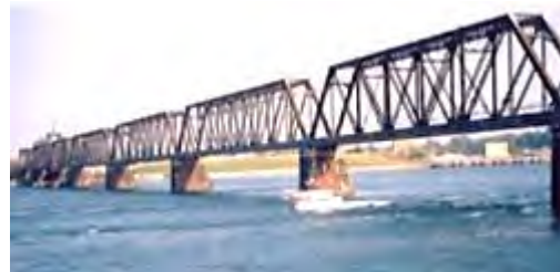
Figure 5-11 International Bridge at Fort Erie, ON
