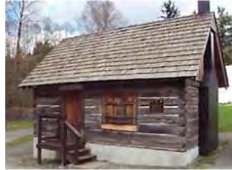
Figure 5-14 Royal Engineer Log Cabin
