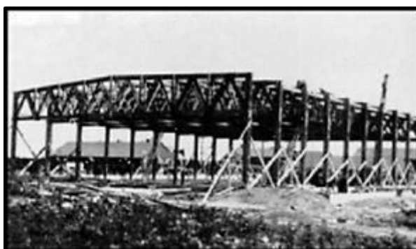
Figure 1-17 Constructing a Hangar for the Air Commonwealth Training Plan
