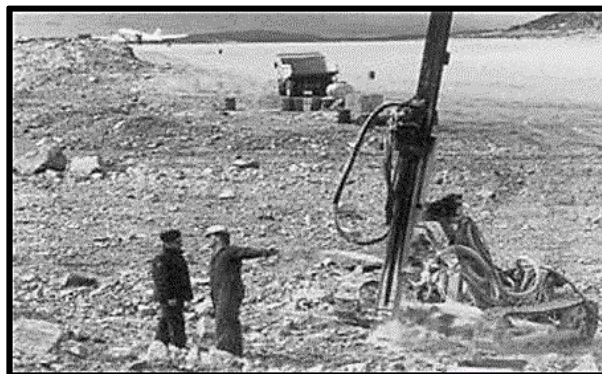
Figure 1-26 Constructing a Northern Airfield
