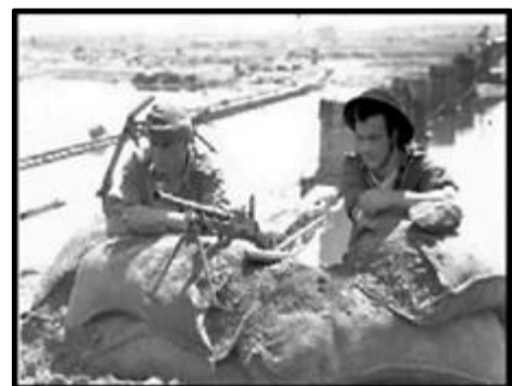
Figure 1-22 Engineers Guard a River Crossing Site in Korea
