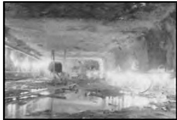
Figure 1-25 Construction of NORAD Control Centre at North Bay
