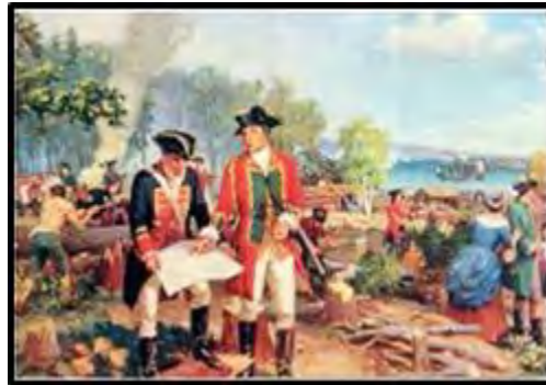
Figure 1-7 Engineers at Work at Halifax
