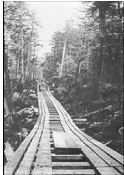
Figure 1-18 CMU Personnel Construct Plank Road to a Remote Site
