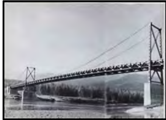
Figure 1-21 Bridge on Alcan Highway
