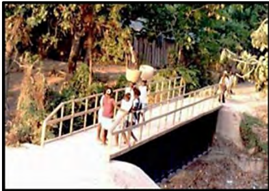
Figure 1-27 Footbridge Constructed in Haiti
