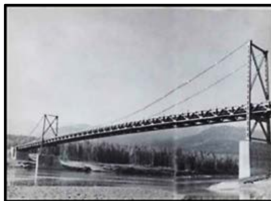
Figure 1-21 Pont de la route Alaska-Canada
