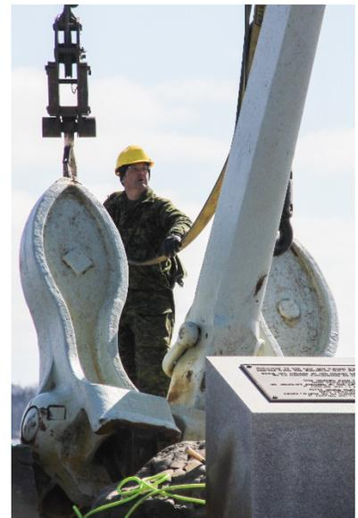
“We came in, moved a lot of the rocks out of the way, disconnected the ship's cable, and freed the anchor from the original mounts and set it off to the side,” Capt Therien said. The team rebuilt the metal supporting structures, replaced the rocks surrounding the monument, and on March 19, moved the anchor back to its original position to be secured to the new mounts.
