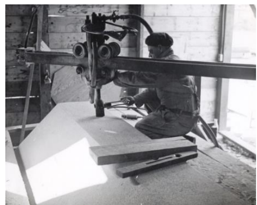
Stonemasons at work
