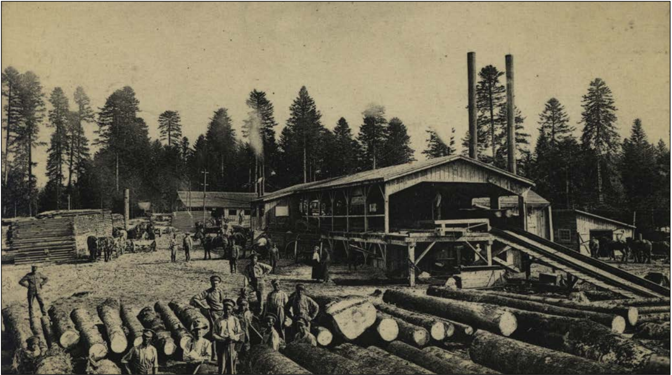
The men of No. 2 Construction Company helped operate the mills of the other forestry companies at La Joux. Note the French lady in the centre of the photo. Local civilians would have been regular visitors to the camp. Note also the horses (far right), the primary source of transportation for the CFC in this area.
