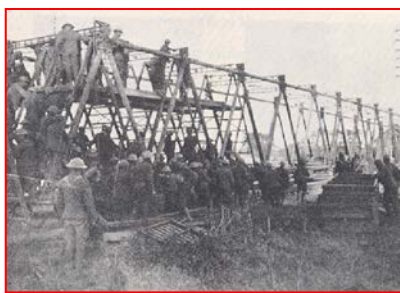
Photo 4 - Inglis bridge under construction, World War I
