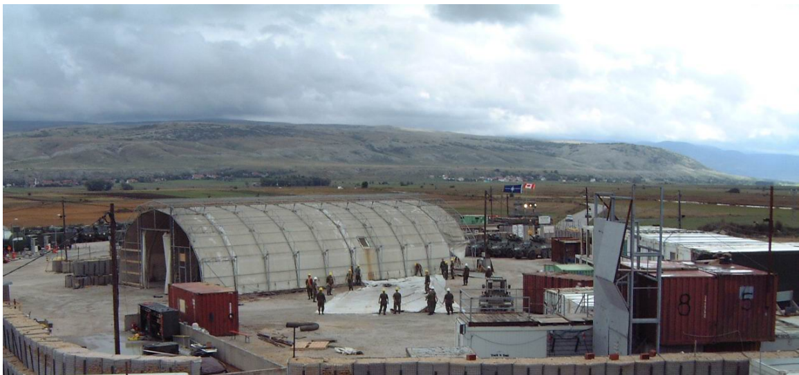
Dismantling of the Maintenance Building (Photographer, WO Demeria, 1 CEU)
