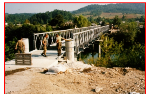
Photo 3 - Bailey bridge deployed in the Former Republic of Yugoslavia
