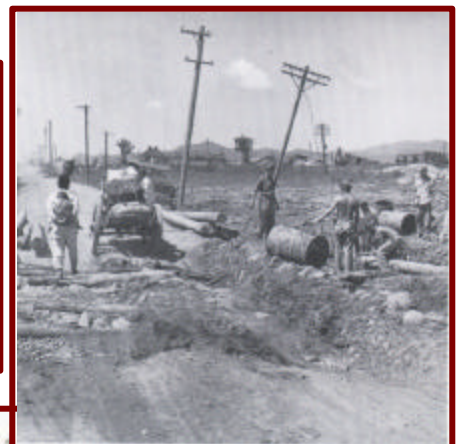
Road repair in Korea, July 1951.
