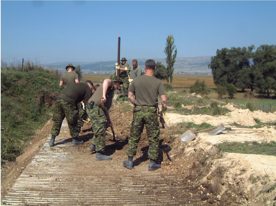
Soil Removal from the TDM (Photographer WO Connolly, 1 CEU)
