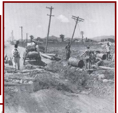
Road repair in Korea, July 1951.
