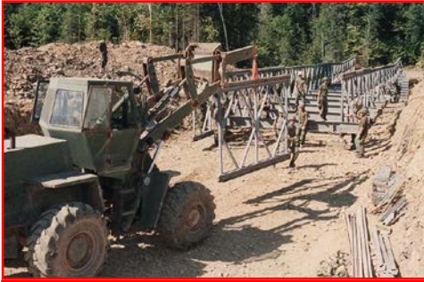
Photo 5 - ACROW bridge under construction
