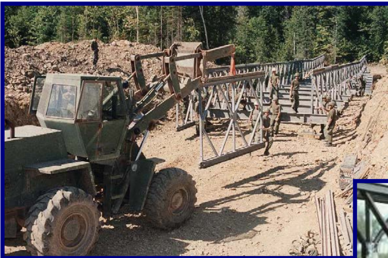
Figure 1 – ACROW under construction using heavy equipment.
