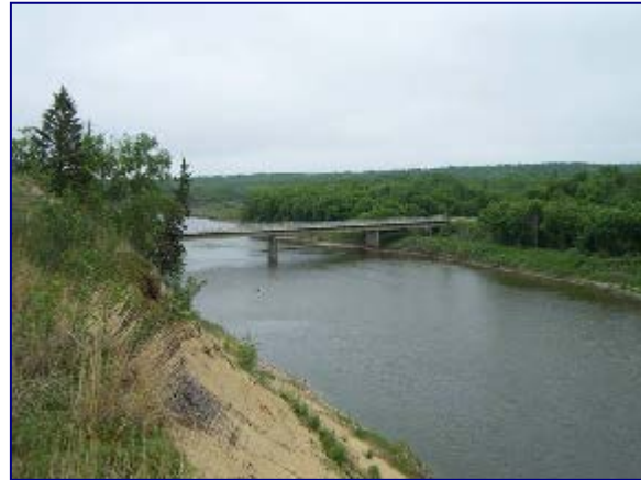
Site of “Bridges for Canada” bridge over the Assiniboine River, MB to be designed and constructed by German military engineers from Pionierbattalion 701, GERA
