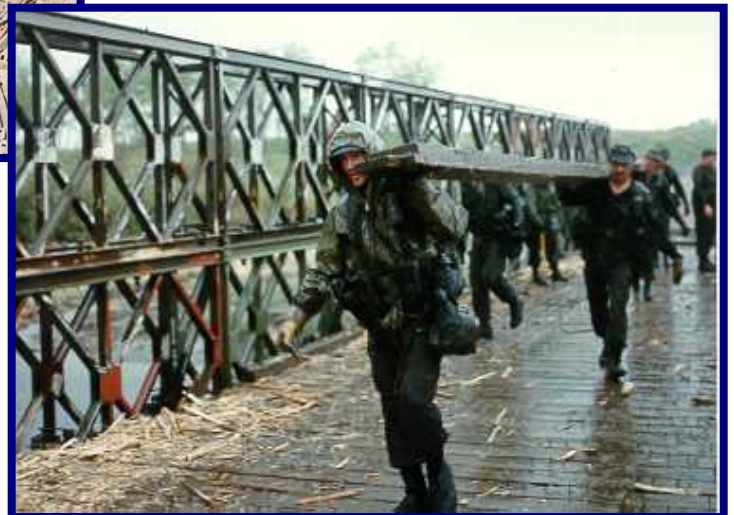
Figure 2 - Bailey Bridge being decked manually.
