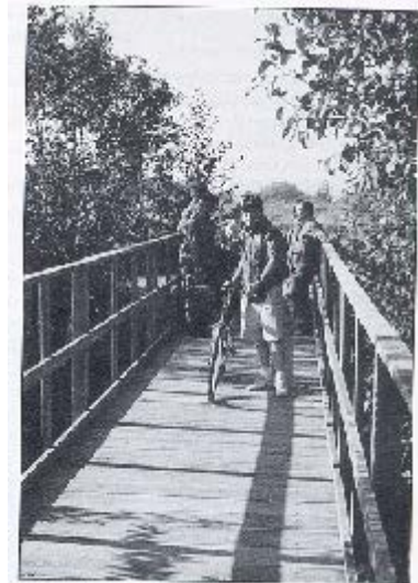
The first crossing of the new span
