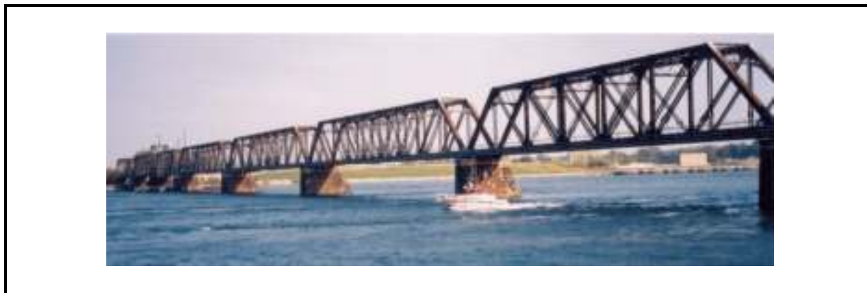
Figure 4-21 International Bridge at Fort Erie, ON
