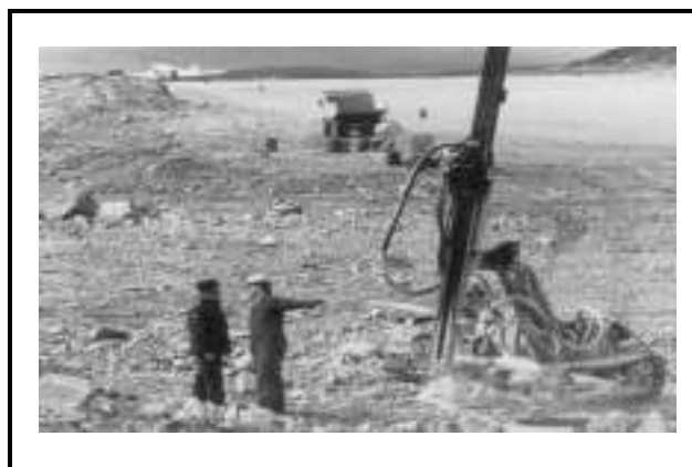
Figure 1-31 Constructing a Northern Airfield
