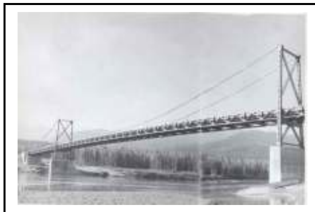
Figure 1-22 Bridge on Alcan Highway
