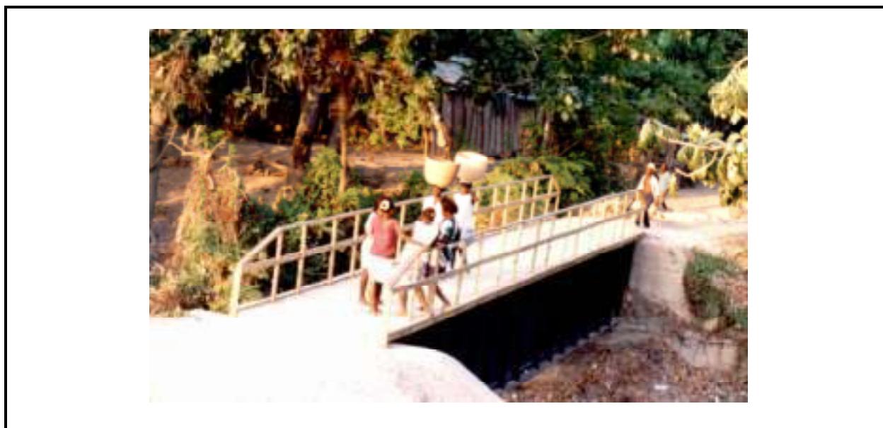
Figure 1-32 Footbridge Constructed in Haiti
