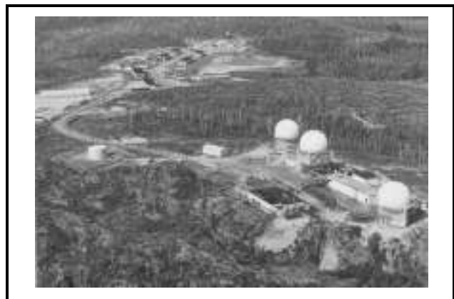
Figure 1-25 Radar Site at Sioux Lookout
