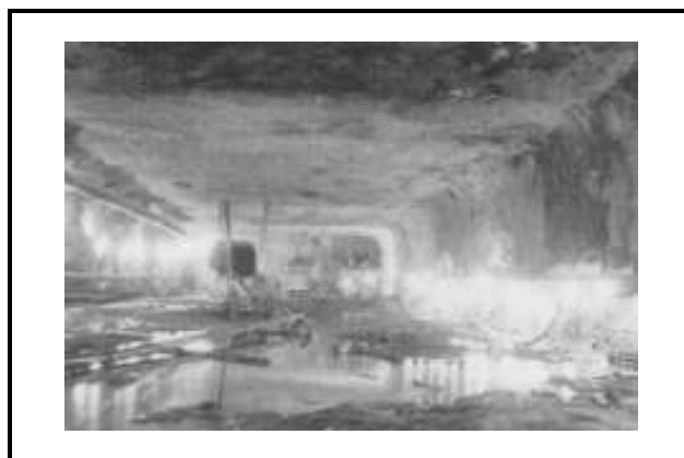
Figure 1-26 Construction of NORAD Control Centre at North Bay
