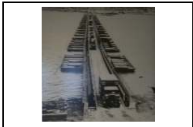
Figure 1-16 Melville Bridge Across the Rhine River
