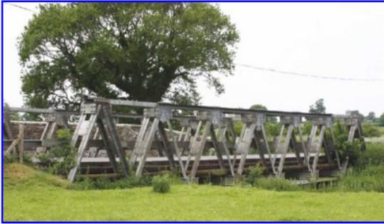
The steel bridge is of the “Unit Construction Bridge” type that was also called the Callender-Hamilton Truss-type bridge. As in other parts of England during WW II, the defence of England against an invasion required upgrading of the local roads and bridges in order to be able to support heavy military traffic like tanks. Taking on such tasks to improve the infrastructure was common for the RCE units that were stationed in England at the time while awaiting the D-Day invasion of mainland Europe.
