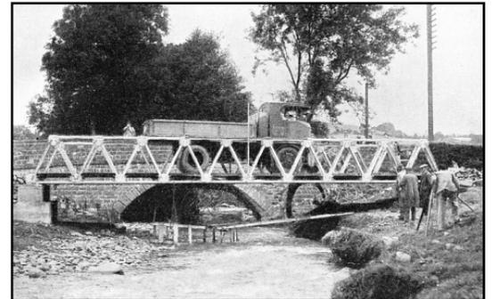
Assembling a Callender-Hamilton bridge took much longer than the Bailey Bridge as it is made up of individual lengths of galvanized steel that are bolted together. It is, however, stronger and simpler in design concept than the Bailey Bridge.
