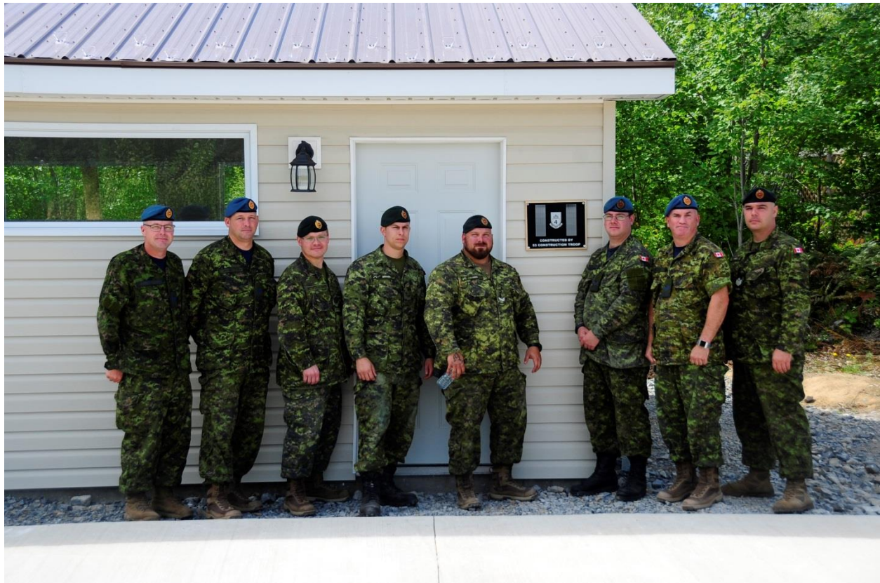
Members of 4 Engineer Support Regiment upon handing over the finished building to the Oromocto Food Bank.
