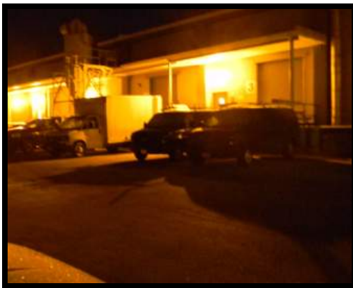
(BLDG P-154 Pre Lighting Retrofit)
