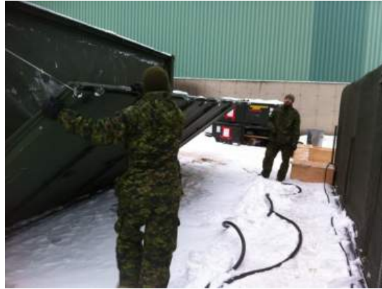
Sgt Leclerc supervises the setup of showers and toilets (MECCs used for ablutions)
