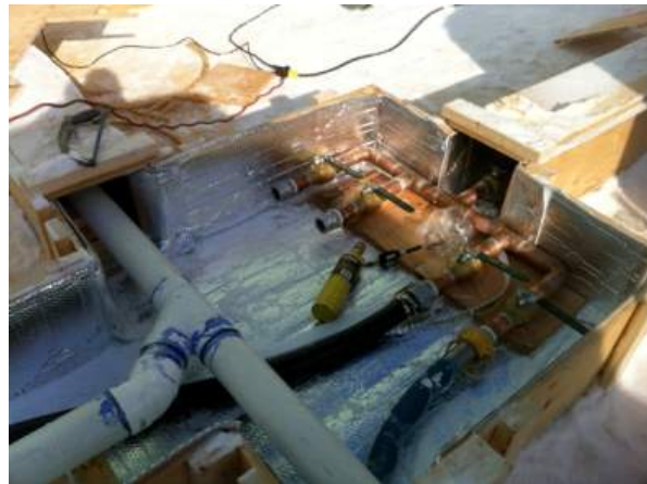
Plumbers design a distribution system for the four MECC Ablutions
