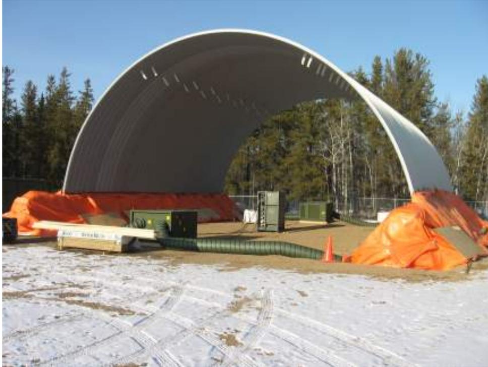
The barrel shaped roof of the practice C-Span, 50' x50', is completed and shown after the pouring of the concrete pony walls which need to be heated and protected from the cold.
