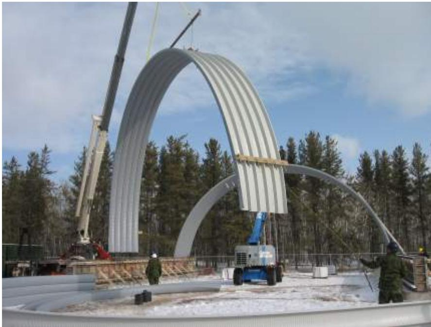
Sheet metal formed and seamed into 5' sections are lifted into position onto a concrete pony wall.
