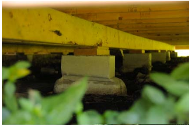
For the sceptics at the time: It seems that you can indeed use an engineer variant of the M113 to build foundation posts. Not an inch of vertical movement over 18 months despite floods and a hurricane.
