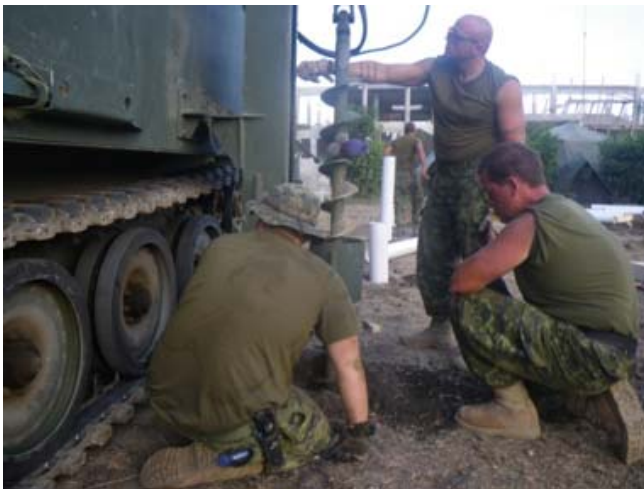
For the sceptics at the time: It seems that you can indeed use an engineer variant of the M113 to build foundation posts. Not an inch of vertical movement over 18 months despite floods and a hurricane.
