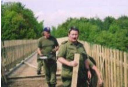
By the end of day two the crew had all posts in place, 95% of the side panels up and 70% of the decking completed. They would have had all the decking completed if they had not run out of lumber on the job-site. Day three saw the crew on site working on the approach "cow catchers" and installing the last side panels and decking. The bridge was completed at 1630 that day.
