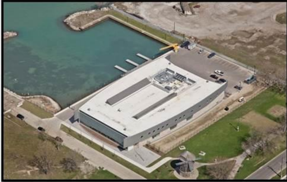
An aerial view of the LEED Gold-certified HMCS Hunter in Windsor, Ontario.
