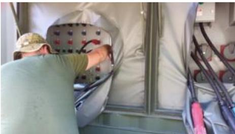
Cpl Buisman, ED Tech, installing the Laundry units to the Power Distribution Unit.
